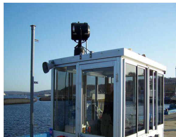
350 Watt Searchlight above at Groton Naval Station Pier
